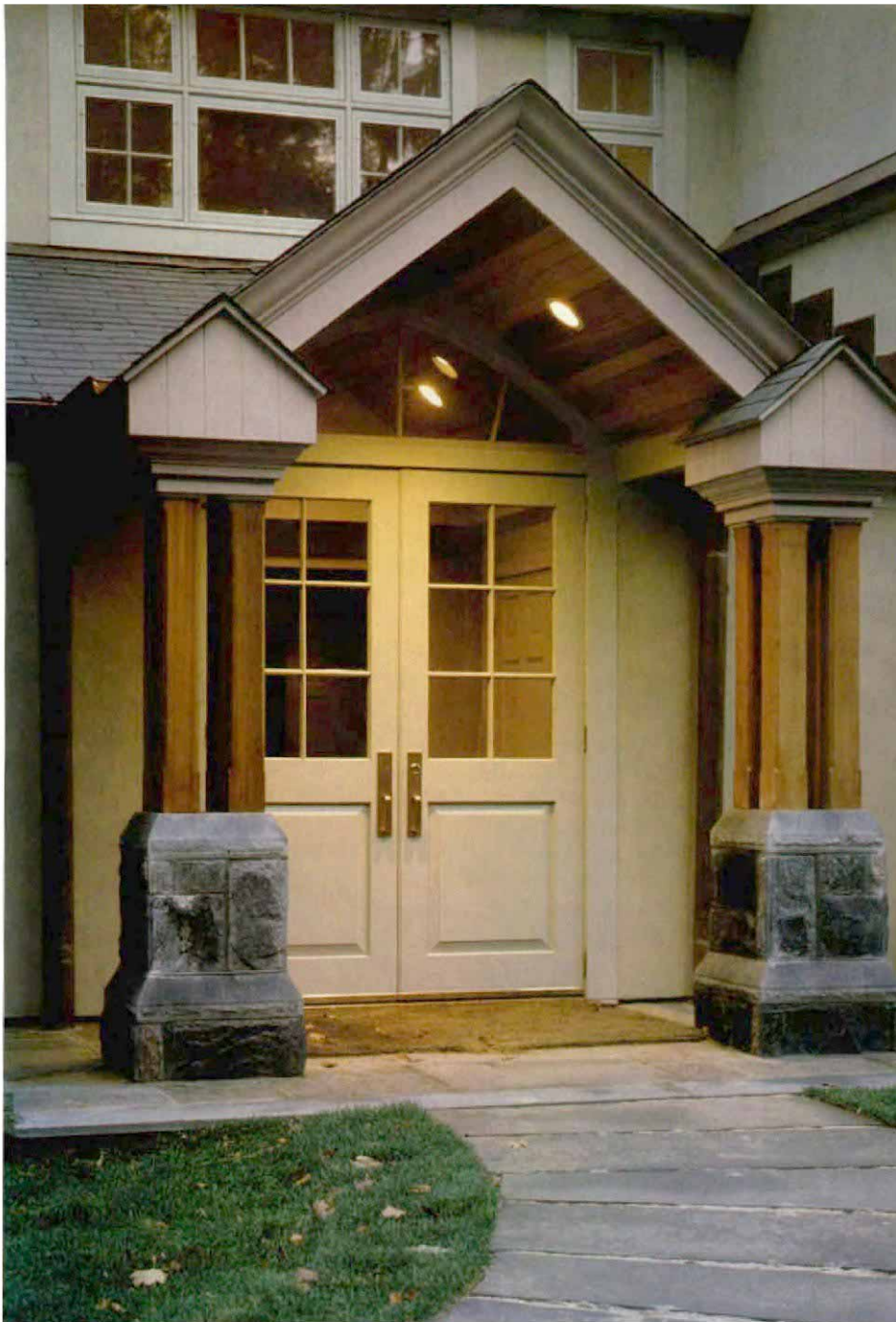
Incandescent fixtures recessed into the porch ceiling warm an entry. A simple arrangement of lights illuminates the doorway and eases the transition between outside and in. Photo courtesy of Phillips Lighting.
